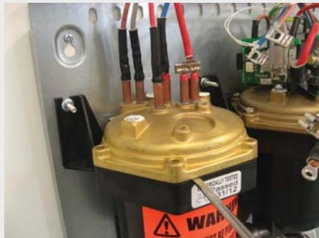
3. Inspect the elements for scale buildup. If scale is present, water supply must be treated to prevent damage to the elements. Consult local water treatment professional for recommendations.
